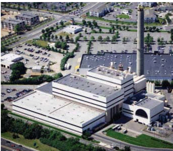
The Hempstead Resource Recovery Facility in Westbury, New York. Environmental excellence will help create community acceptance of WTE facilities. PHOTO: COVANTA ENERGY CORPORATION
